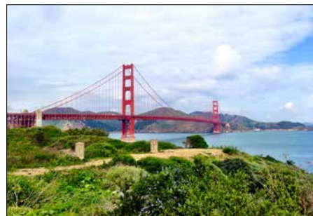
Golden Gate Bridge, San Francisco
